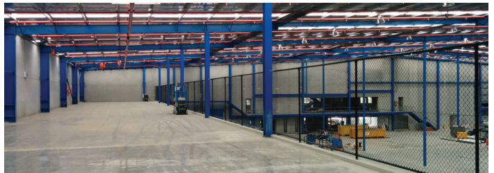
Mezzanine deck 3PL area
